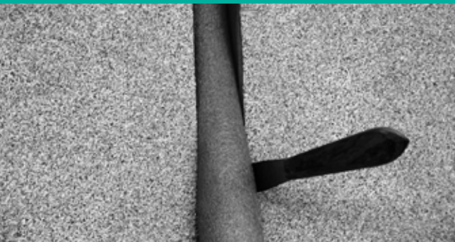
FIGURE 7.1 – INSERTING BACKER ROD
